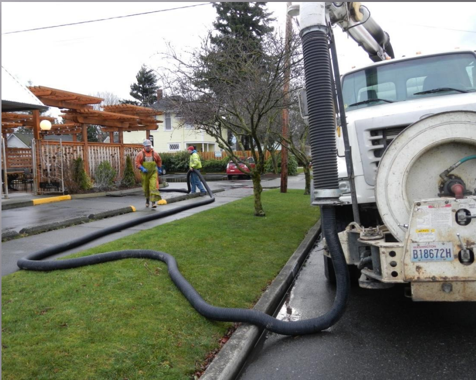
Vactor truck cleaning out catch basins
