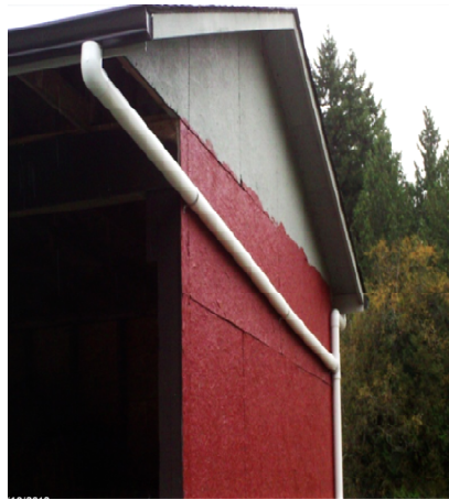
Gutters and downspouts
