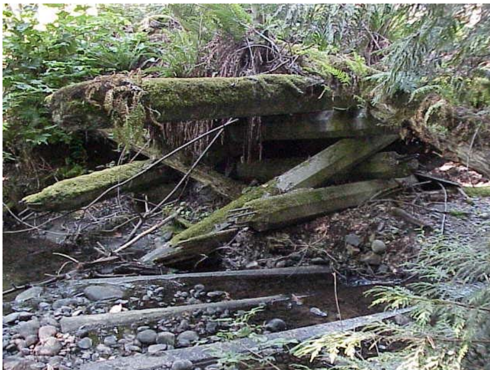
Impromptu Bank Armoring, Carpenter Creek
