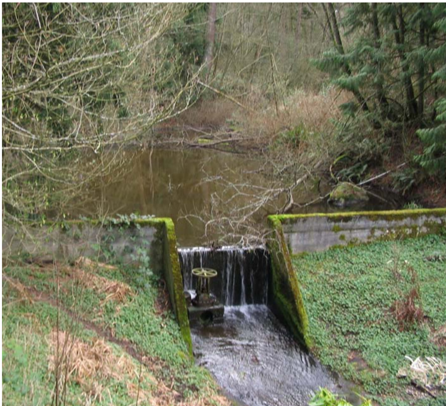
Private Dam above County Line Road/332 St. NW, Little Fisher Creek
