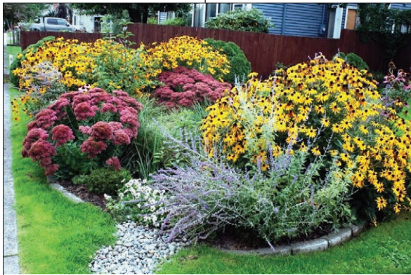
Rain gardens are versatile features that can be installed in almost any unpaved space. Also known as bioretention, or bioinfiltration, cells, they are shallow, vegetated basins that collect and absorb runoff from rooftops, sidewalks, and streets. This practice mimics natural hydrology by infiltrating, and evaporating and transpiring—or “evapotranspiring”—stormwater runoff.
