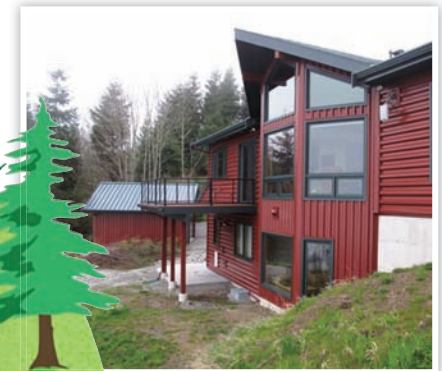
Above: This house features Firewise construction concepts such as a metal roof and non-combustible siding.
