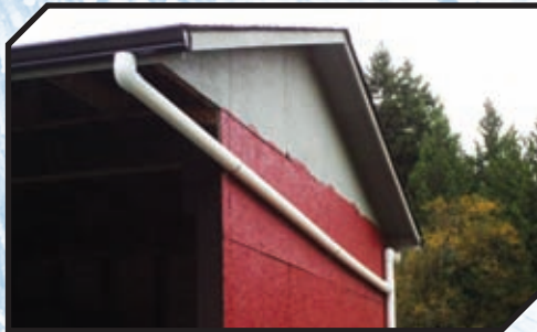
Gutters and downspouts
