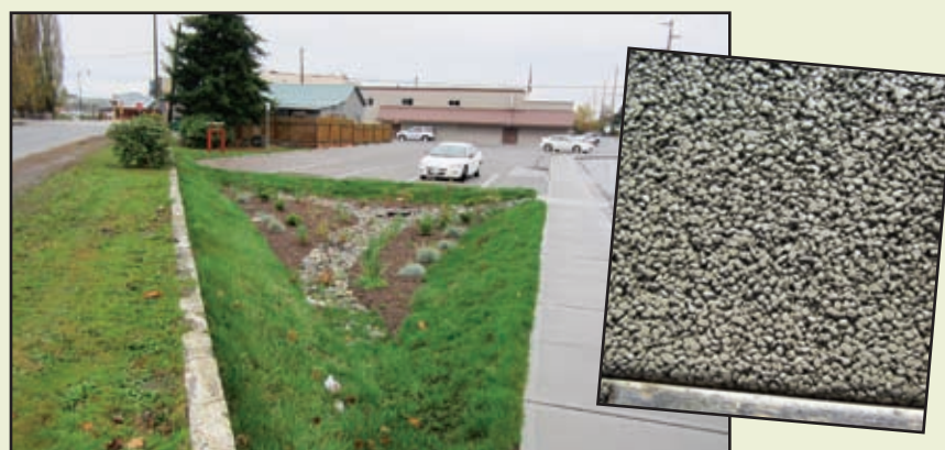
The Victoria Ave. LID project includes a rain garden and a new porous paved parking lot. Porous pavement stores and infiltrates surface runoff, increasing groundwater recharge and reducing pollution.
